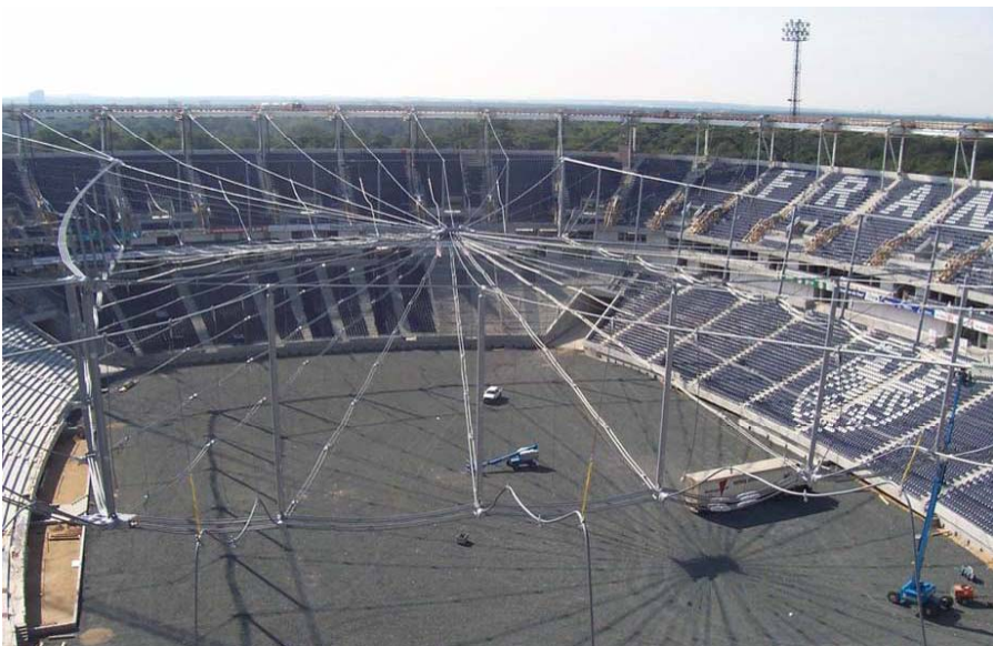
▼ The cable net at the end of the first stage with the flying masts installed
