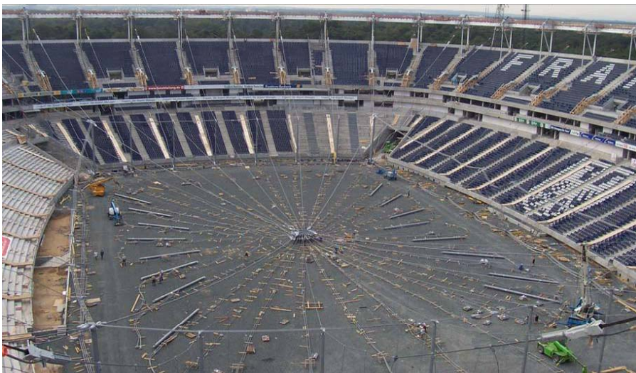
▼ The cable net at the end of the first stage with the flying masts installed
